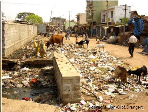
Animals scavenging organic material and clogged storm water drains
