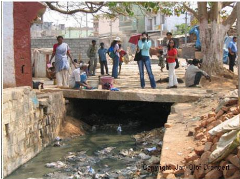
Stormwater drainage as a conduit for solid waste
