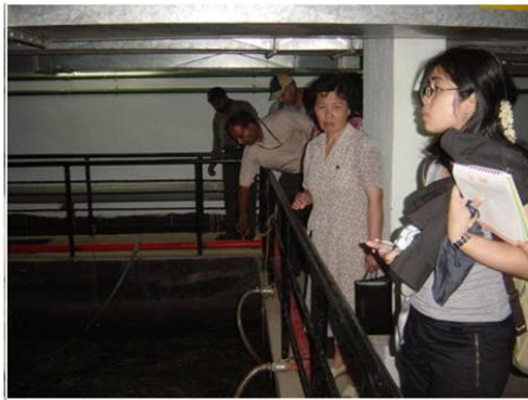
Sedimentation and aeration tanks
