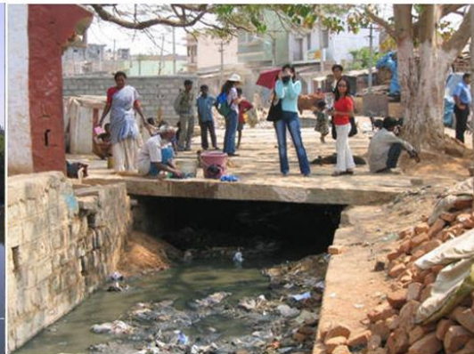
Wastewater and stormwater drainage in Bangalore, India
