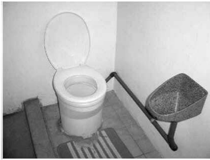
a) Urine-diverting pedestal in plastic, South Africa
