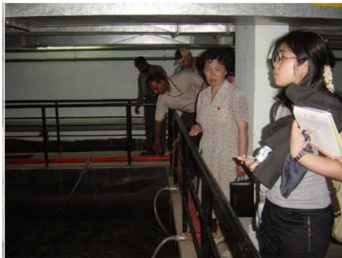
Sedimentation and aeration tanks
