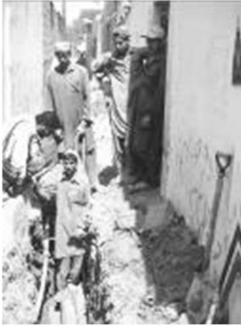
Digging for sewers in Orangi
