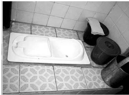
b) Urine-diverting squatting pan in fibreglass, China
