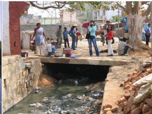
Wastewater and stormwater drainage in Bangalore, India
