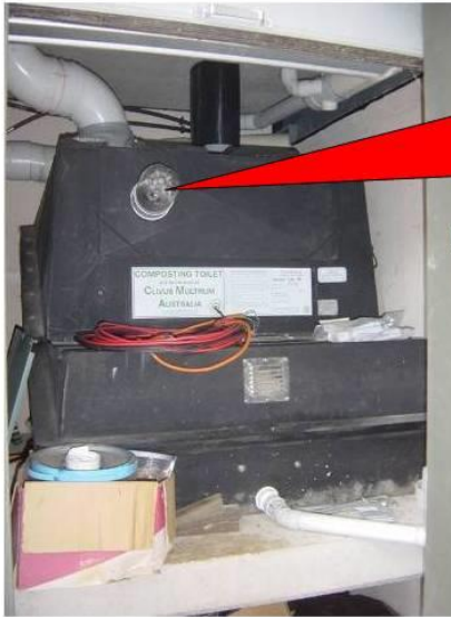
Newly installed container for excreta (Clivus Multrum)
