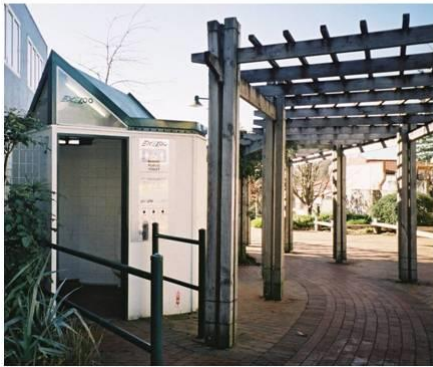
Excellent access to unisex street toilets in Waikato, New Zealand.
