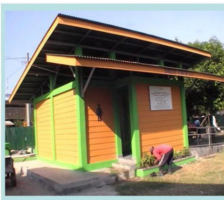
Girls' school toilet, Indonesia with natural light and ventilation
