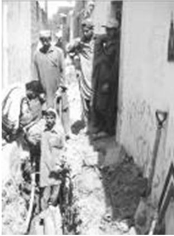
Digging for sewers in Orangi
