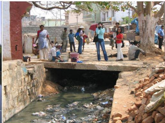
Wastewater and stormwater drainage in Bangalore, India
