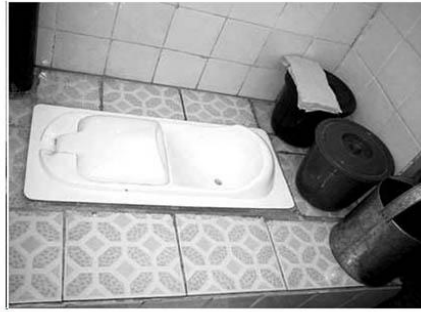
b) Urine-diverting squatting pan in fibreglass, China
