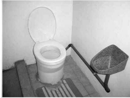
a) Urine-diverting pedestal in plastic, South Africa
